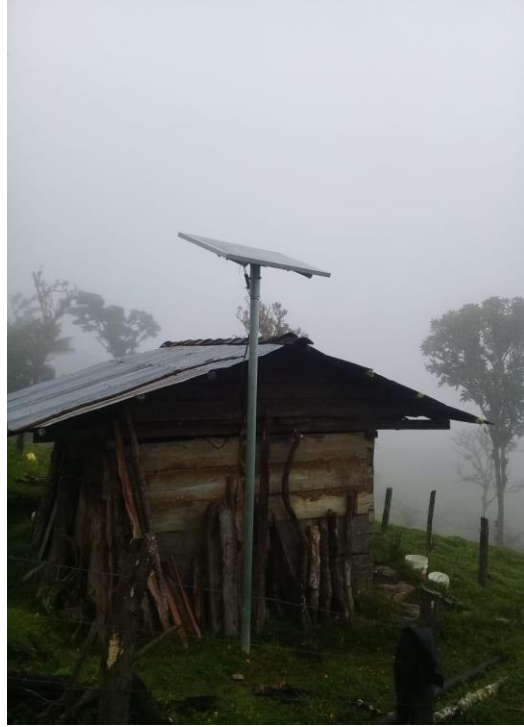
Figure 14 Casa de Campo, farm house, with newly installed solar panel
